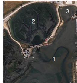
Figure 15- Aerial view of the lagoon system.
